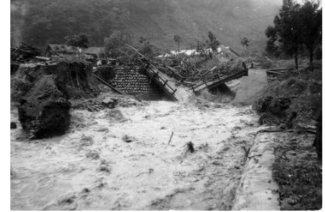
護岸の破壊と橋梁の落下
